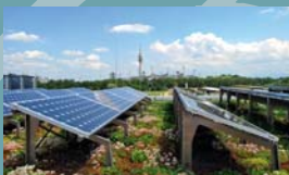
Green Roofs + Photovoltaic, MTZ Munich; Germany
