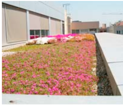
Extensive Green Roof in Barcelona
