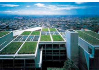
Extensive Green Roof
