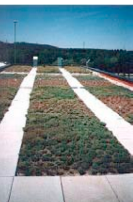
Green Roof at the Plant Production Pavilion, E.T.S.I.A, Madrid
