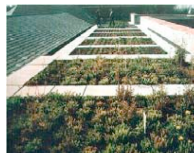
Green Roof at the Department of Economics, E.T.S.I.A, Madrid
