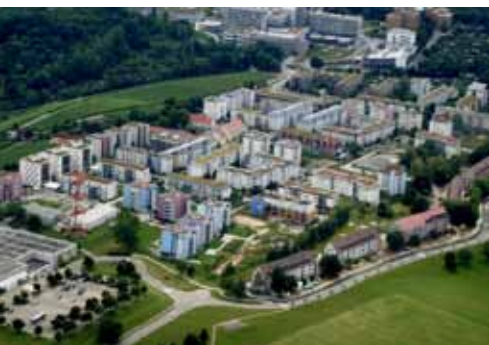
The aerial view demonstrates the success of the green roof policy in Germany
