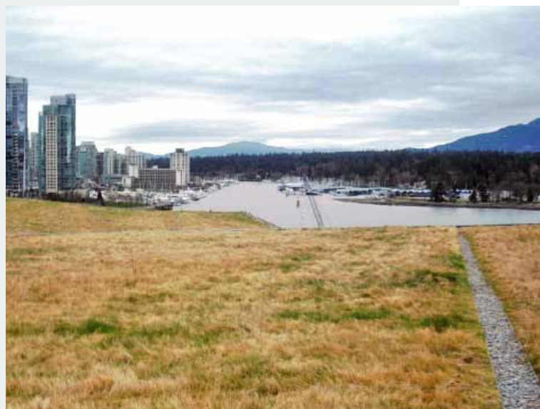
The Vancouver Convention Centre roof in March 2011
