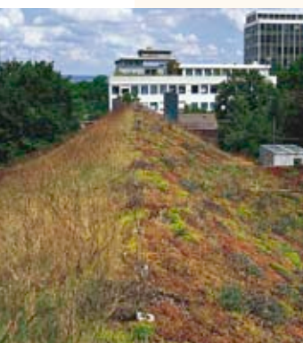
Different plant communities on a ridged roof (left side: north exposure, right side south exposure)
