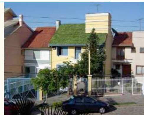
Modular light-weight system Ecotelhado allows installing 120 sqm in one day.
