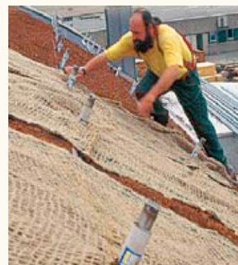
Additional protection with anti-erosion net for pitched roofs > 15°
