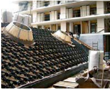
Georaster - stable grid element for steep pitched roofs
