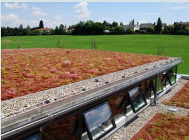
Thermally insulation with green roofs
