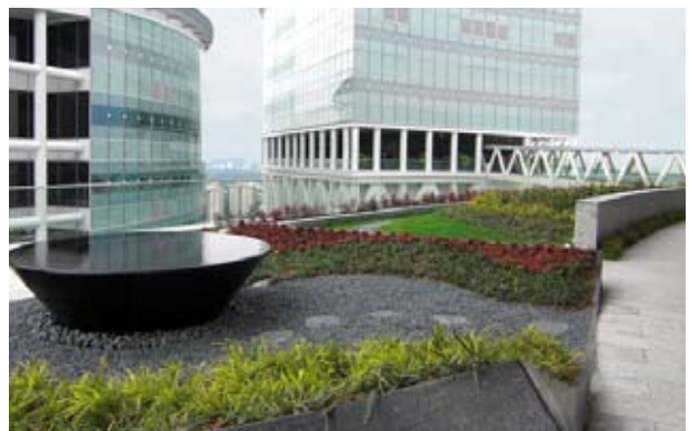
The roof gardens of Fusionopolis serve as the green lungs and social pockets for the office and lab staff. Courtesy: ZinCo Singapore Ltd
