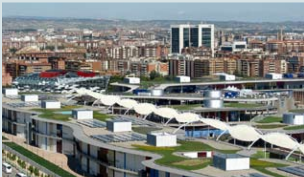
The green roofs on top of the "Pavillones de las Naciones" at the EXPO 2008 in Zaragoza.
