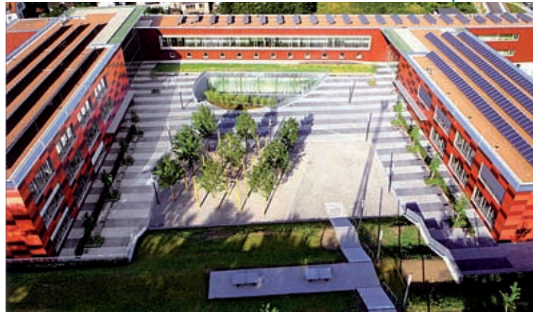
Sustainability and education: Germany's latest educational centre in "Passivhausstandard" also features a combination of green roofs and photovoltaics
