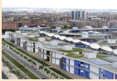
The looping rooftop landscape of the 'Pavilion of Nations'
