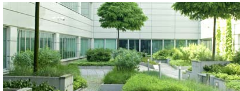
Recreational Roof Gardens – landscape design by Dorota Rudawa
