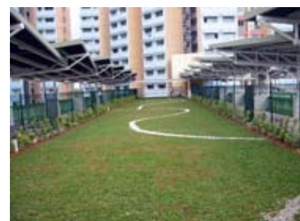
The existing old MSCP was transformed into a roof garden for the public's enjoyment.
